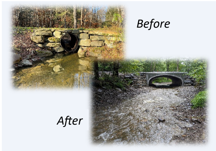
Corbin Creek- Warren Twp Culvert Replacement
