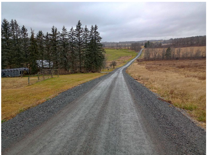
On this project tree removal provided room to establish a Flexamat stabilized ditch along the right side of the project, while establishing sheet flow on the left. Banks were sloped gently enough to allow for easy mowing to provide low-cost maintenance as well. We were also able to utilize an existing diversion swale to break up runoff from the project thanks to landowner cooperation.
