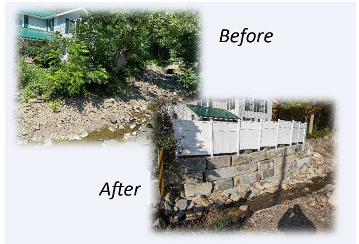
Golf Creek- Granville Twp Stream Bank Restoration
