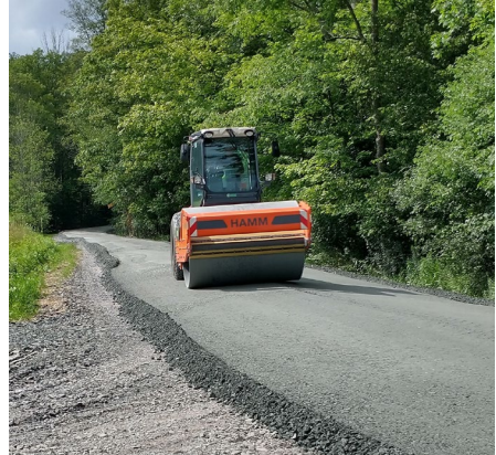
After: final surface placement at end of dirt work.
