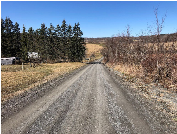
On this project tree removal provided room to establish a Flexamat stabilized ditch along the right side of the project, while establishing sheet flow on the left. Banks were sloped gently enough to allow for easy mowing to provide low-cost maintenance as well. We were also able to utilize an existing diversion swale to break up runoff from the project thanks to landowner cooperation.
