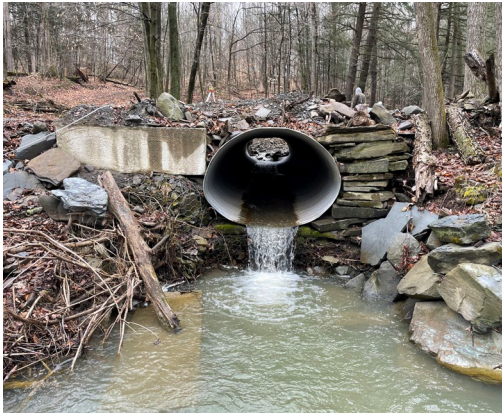
Before: Large scour pools, undersized culverts, ditch scouring and large deposits of sediment from flood damage.
