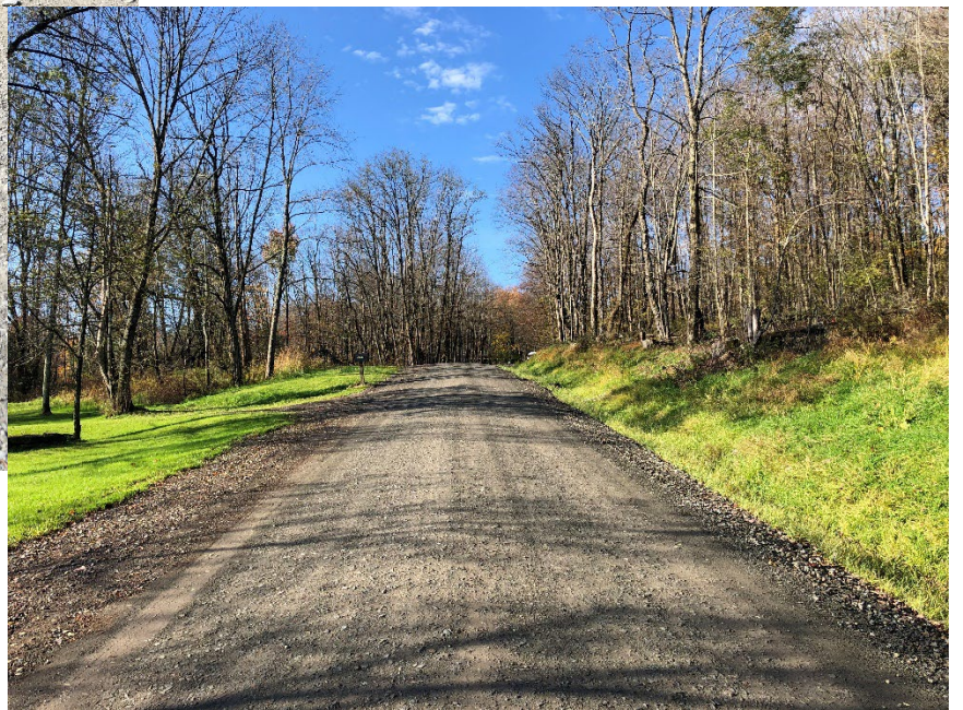
Road fill to allow sheet flow.
